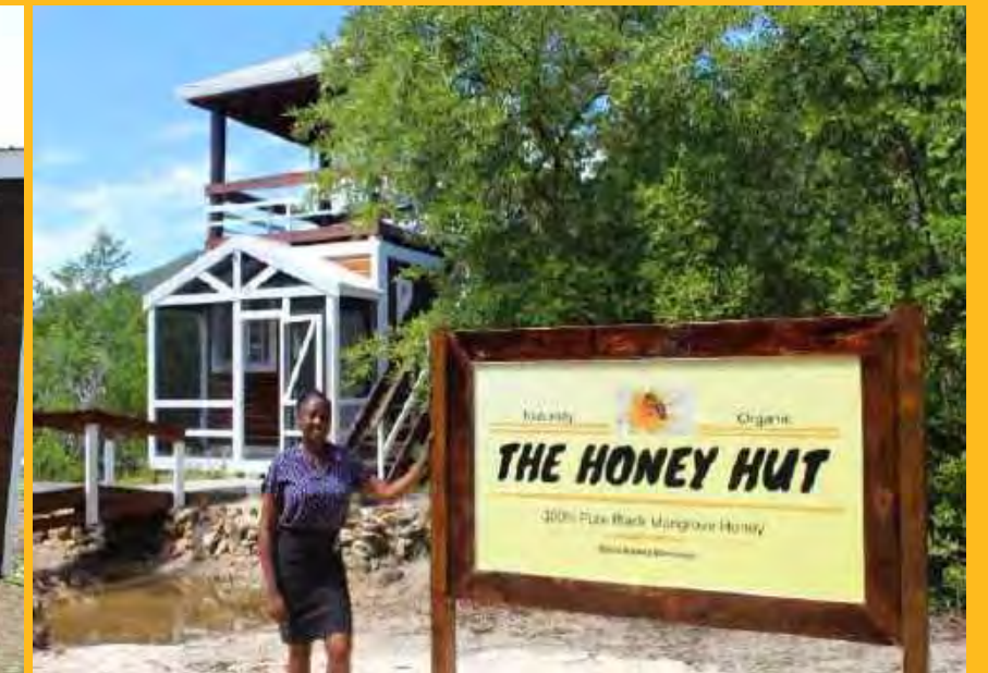
Constructed honey facility in St Vincent and the Grenadines
