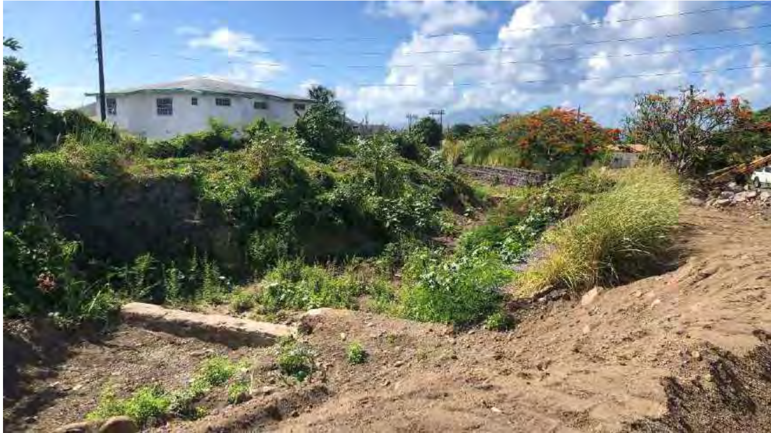
Land Degradation Control Works College Street Ghaut
