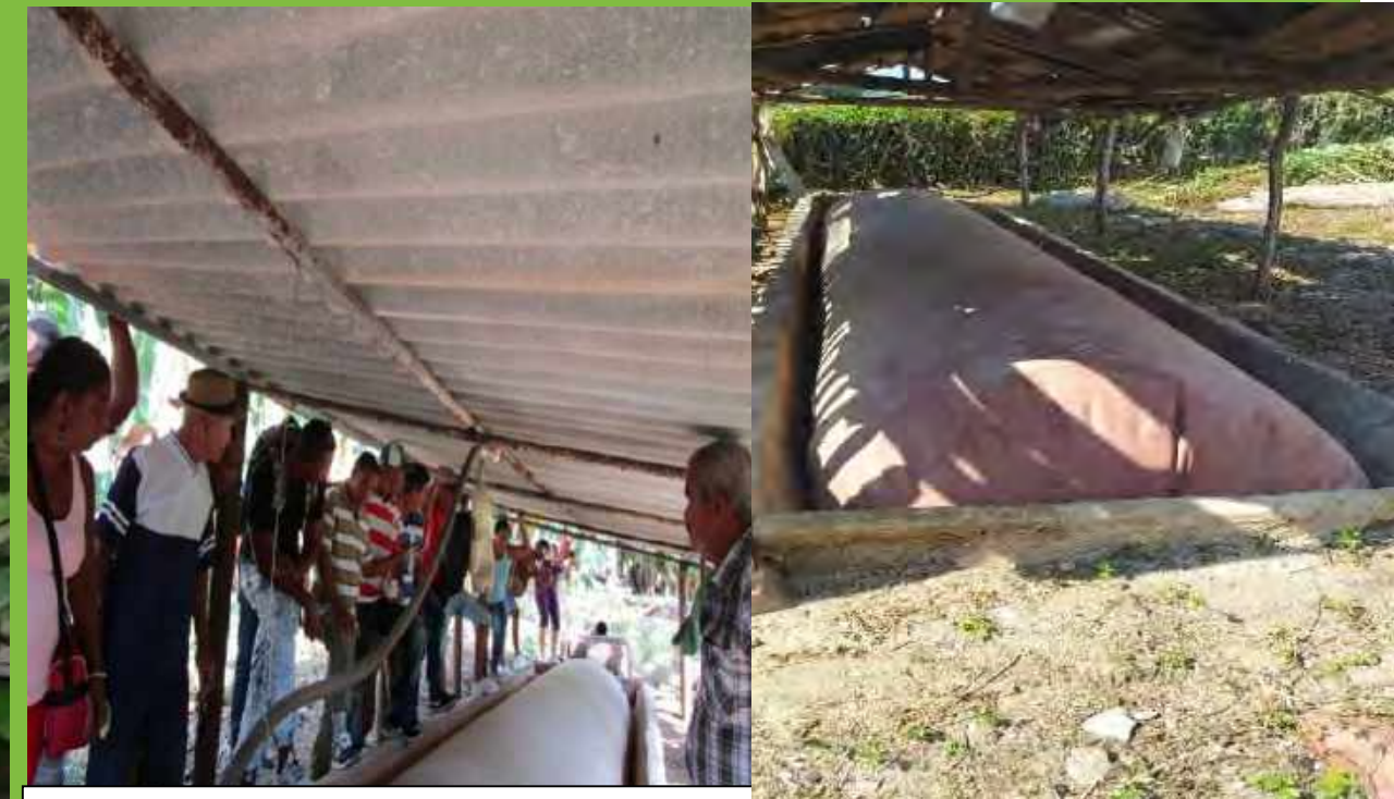
A demonstration training workshop for the installation of a 10 cubic meter geomembrane tubular biodigester on a farm.
