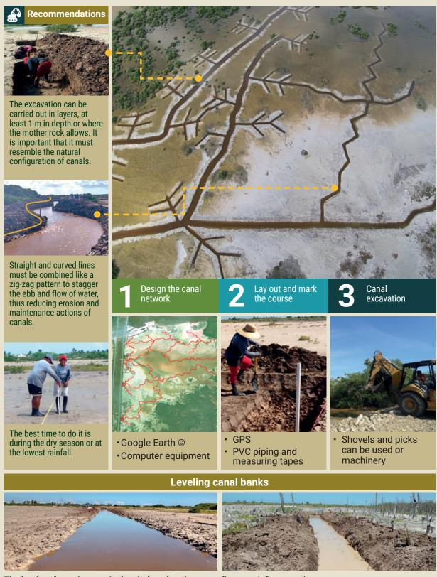
The banks of canals must be leveled so that the water flow can influence a larger area.
