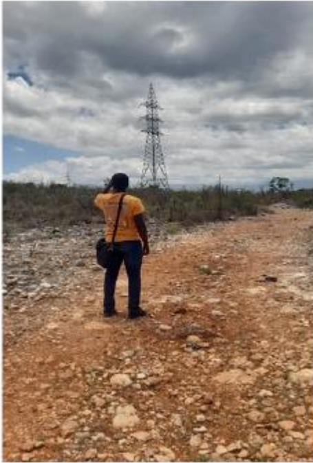
Measuring height of power line tower with height meter
