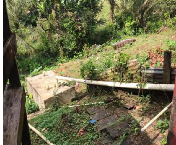
Figure 9: Household connected to a Lined Pit (Source: Rabicia/EPA./2022).
