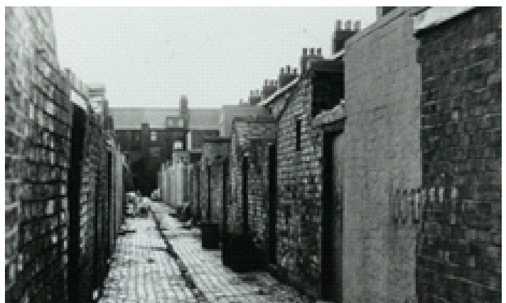
Figure 7: Terraced housing in London with outdoor toilets – the collector sewer ran down the back of the houses.
