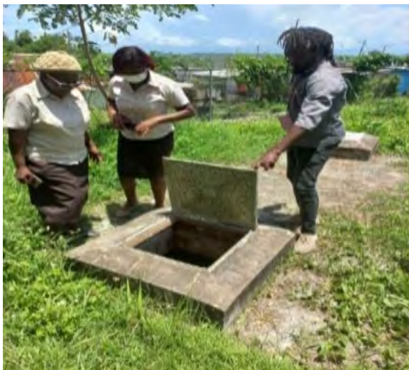
Figure 9: STs connected to soak pit (Source: Jodian/Org./2022).
