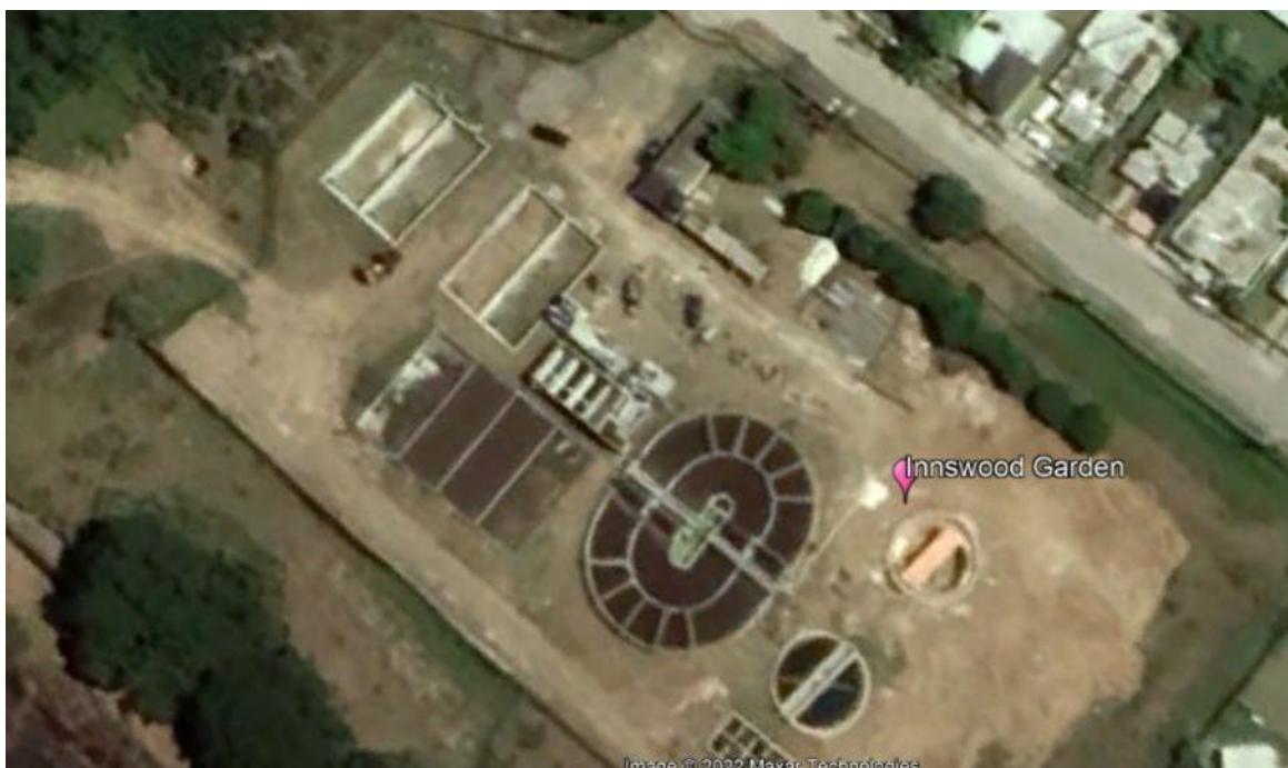
Figure 1 - Innswood garden Oxidation ditch
