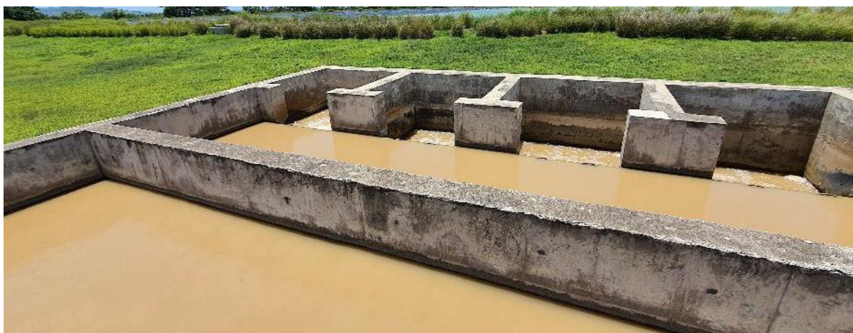
Figure 3 - Aquifer recharge Innswood – inlet to the plant with water from the canal
