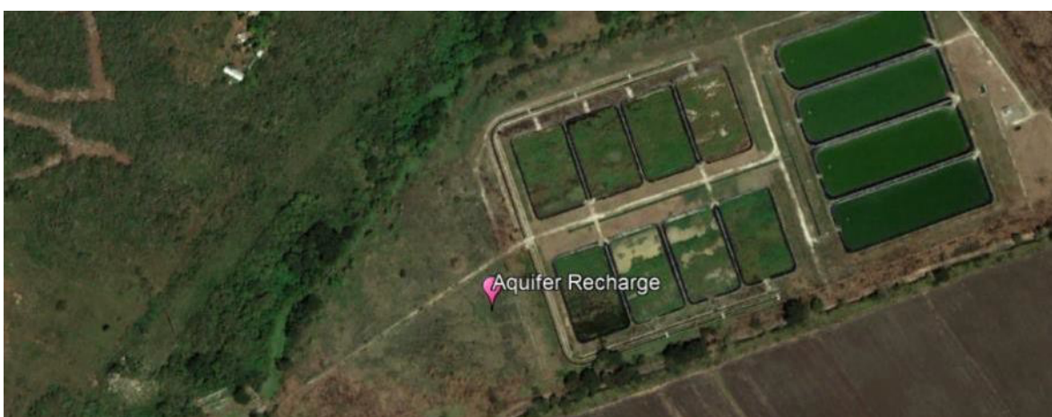
Figure 2 - Innswood - Aquifer Recharge facility
