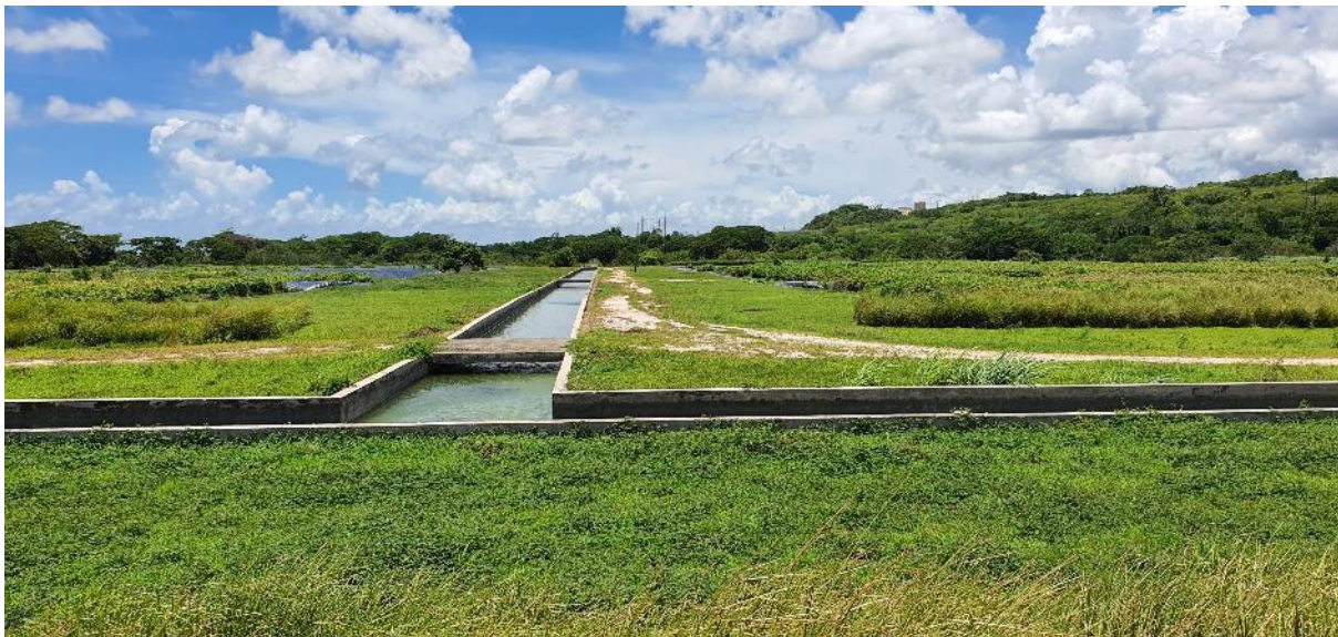
Figure 5 - Aquifer recharge Innswood – reed beds
